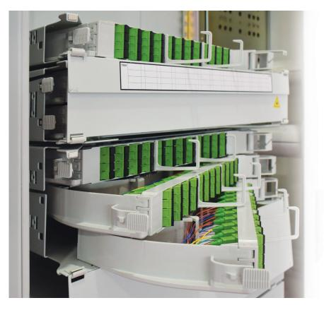
FOCUS NPTD subracks can be mounted on **ETSI** frames by using suitable brackets. Please, contact our offices for more info.
